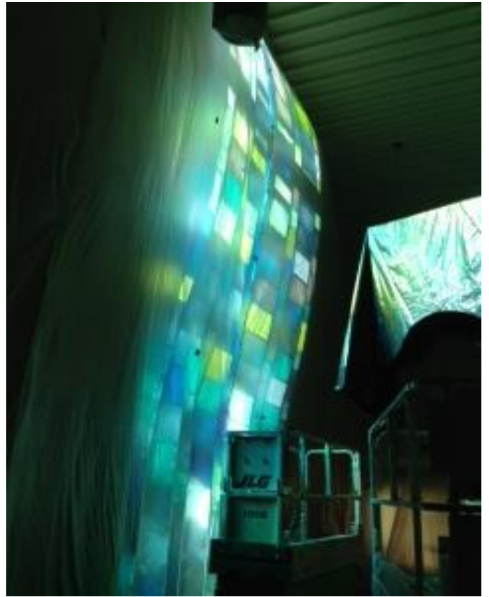
Stained glass window covered up while the painters worked.
