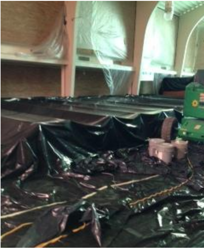
Sanctuary pews and walls covered with plastic.
